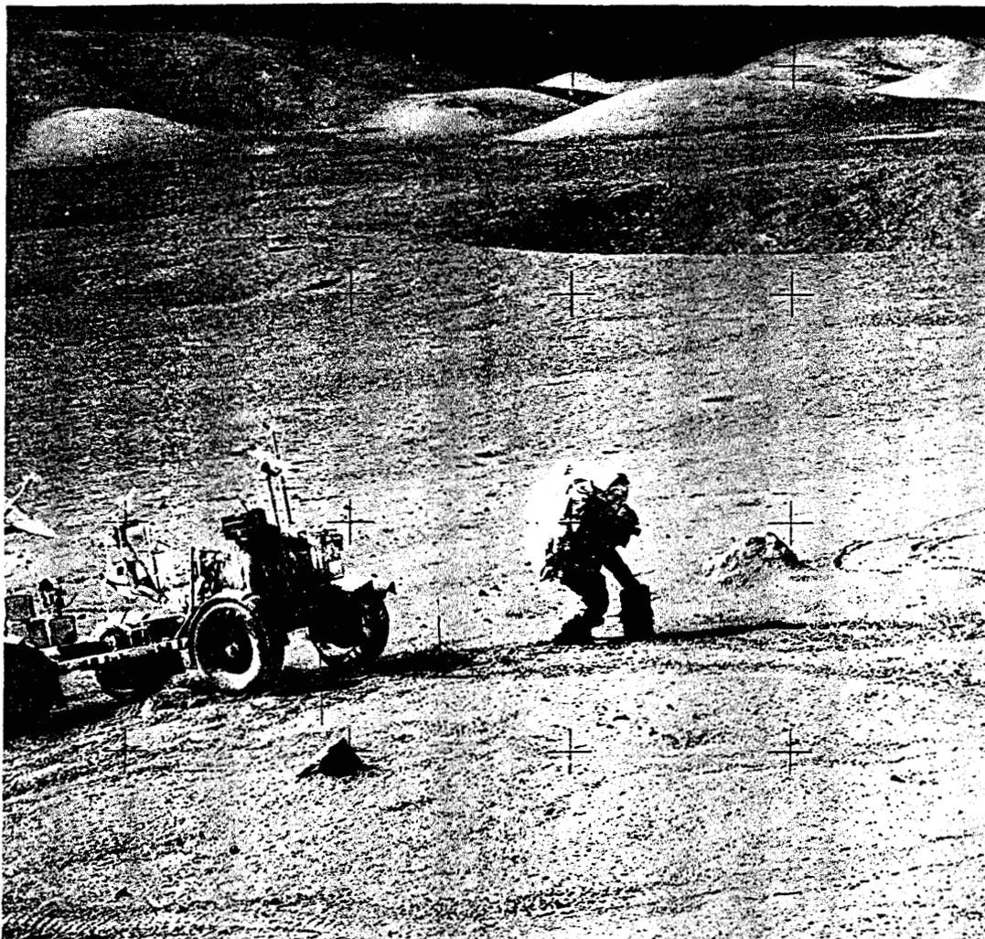
Figure 10-16.- Commander place the traverse gravimeter on the lunar surface.
